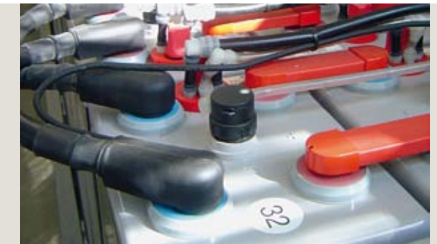
Storage technology New reserves for power grids
