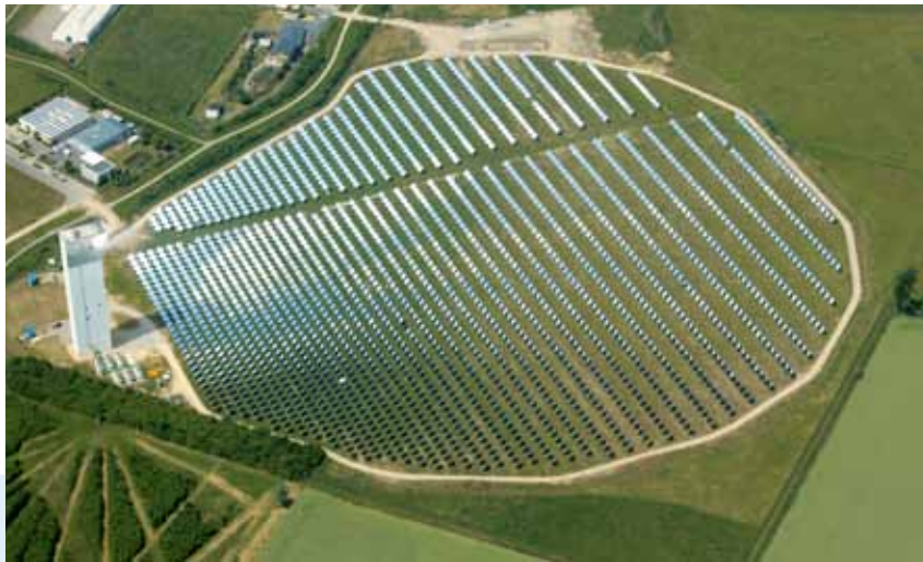
The solar tower in Jülich is allowing DLR experts to develop and test innovations in solar thermal power generation more quickly and on a real-life scale. Photo: DLR
