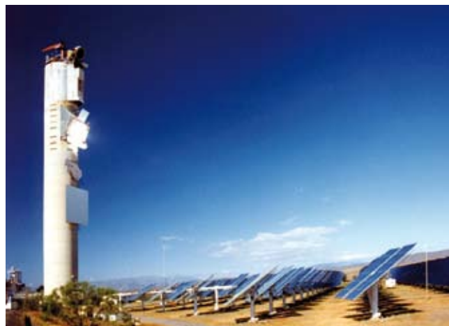
THE SOLAR POWER STATION TOWER ON THE PLATAFORMA SOLAR IN ALMERÍA IS SURROUNDED BY A MIRROR ARRAY THAT FOCUSES THE SUNLIGHT ONTO THREE RADIATION RECEIVERS. A SOLAR-HYBRID GAS TURBINE IS LOCATED WITHIN THE TOWER. Photo: DLR
