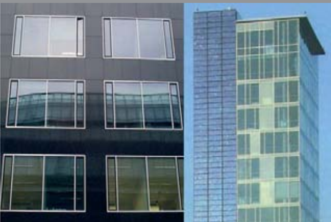
FACADES FITTED WITH BLACK CIS MODULES (LEFT, AS A MODEL) WOULD LOOK AS ELEGANT AS THIS. NEXT TO IT A FACADE WITH CONVENTIONAL SOLAR CELLS. Photo: Nikolaus Meyer
