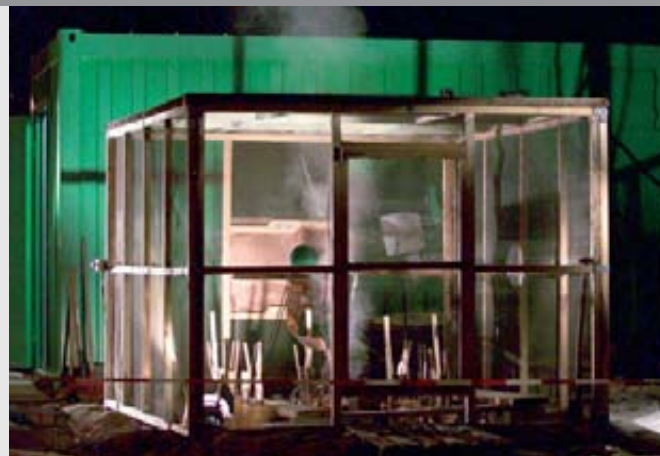
THE RADIOWAVE-BASED SOIL REHABILITATION TECHNOLOGY WAS SUCCESSFULLY TRIED OUT AT LAB, PILOT PLANT AND FIELD SCALE. Photo: UFZ/André Künzelmann
