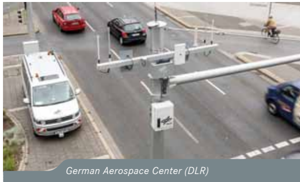
Test intersection in Braunschweig. Photo: DLR (CC-BY 3.0)
