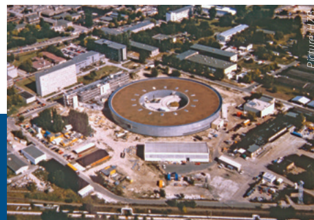
After only four years' construction time, BESSY II is complete. The ceremonial commissioning takes place in September – a spark that sets off the development of Adlershof.
