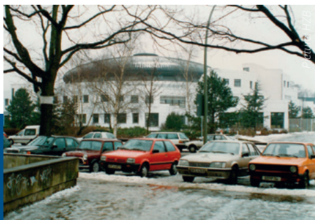
The location of BESSY I in Berlin-Wilmersdorf is simply too small. With German reunification comes the opportunity to rebuild in Adlershof.
