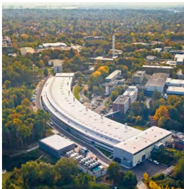
THE AERIAL PICTURE SHOWS THE PETRA III EXPERIMENT HALL THAT IS 300 METRES LONG AND HAS ROOM FOR 30 NEW EXPERIMENTS. Photo: DESY
