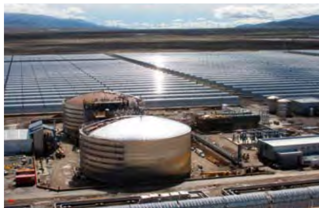
ANDASOL 1: 520,000 SQUARE METRES OF MIRRORED SURFACE CAPTURES THE SUNLIGHT. Photo: Solar Millenium AG
