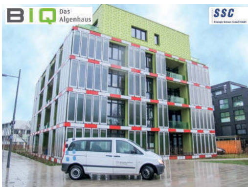
Algae grow inside the facade, nourished by CO 2 from the building's heating system. Image: HZG
