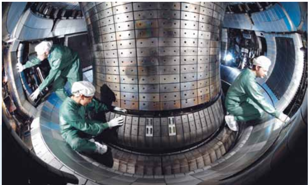
Installing control coils in the plasma vessel of the ASDEX Upgrade fusion device. Photo: IPP/V. Rohde
