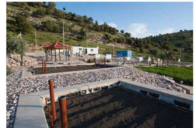
Research and demonstration facility in Fuheis (Jordan) to analyse treated wastewater and flood water, and to work on capacity development measures. © André Künzelmann, UFZ
