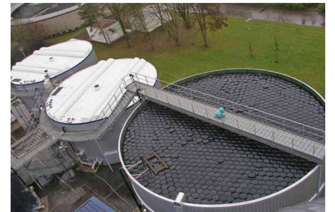
Deammonification reactor for treatment of process water in the main wastewater treatment plant in Ingolstadt. © N. Wagner, KIT
